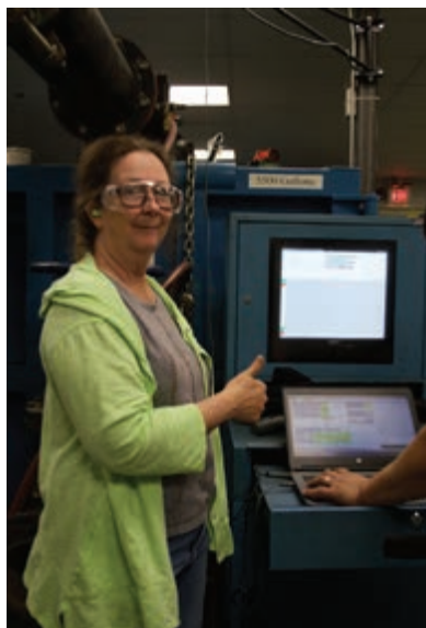
LeEllen Phelps, NSO Thermal Systems Manager, signals that the pumps passed all required factory-acceptance tests.
