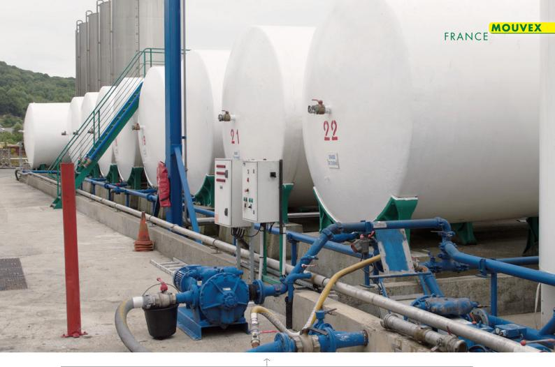
France-based Olvea Group is supplying fish, lard and vegetable oils for food production; and helping them along the way have been A Series and P Series Eccentric Disc Pumps from Mouvex.
